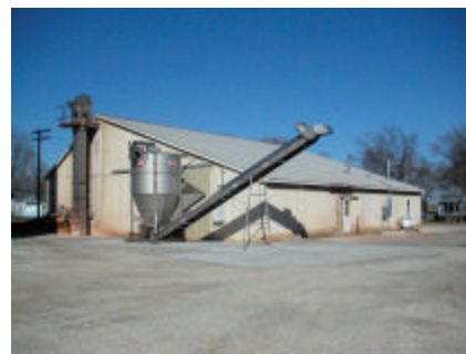
Lenzburg Fertilizer Plant P.O. Box 297 116 E. North Railroad Lenzburg, IL 52255 (618) 475-3228
